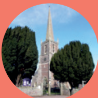
WINTERBOURNE PARISH CHURCH
